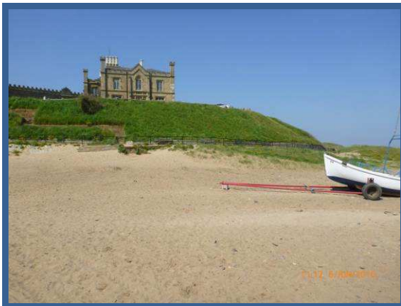
Vegetated slope above masonry wall CBU E52/7
