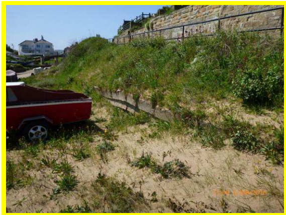
High beach levels and vegetation cover obscuring masonry wall and revetment north west of beach entrance (/C0702C01)
