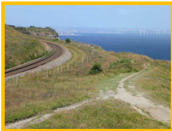
E54/3a proximity of footpath and railway line to actively eroding cliff top (Partly Active)
