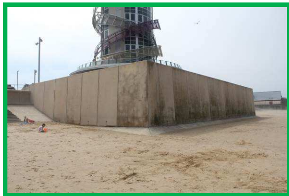
Concrete sea wall at Redcar Beacon (/C0602C03)
