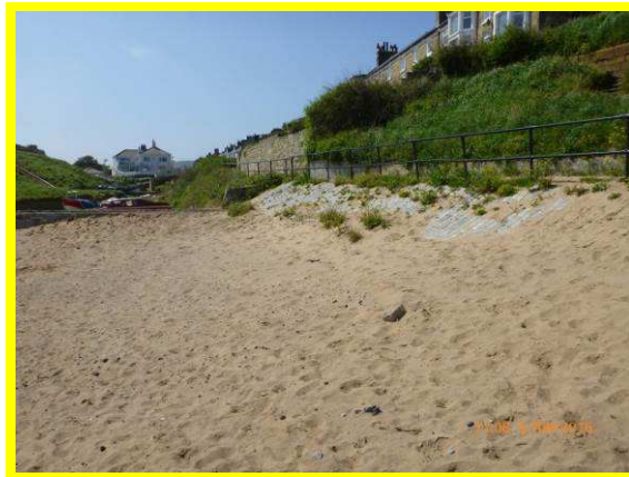
High beach levels and vegetation cover obscuring masonry wall and revetment north west of beach entrance (/C0702C01)
