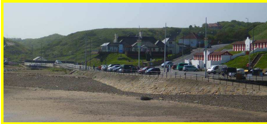
View looking southeast from pier. Beach levels lower at 'apex' of headland (/C0704C01)
