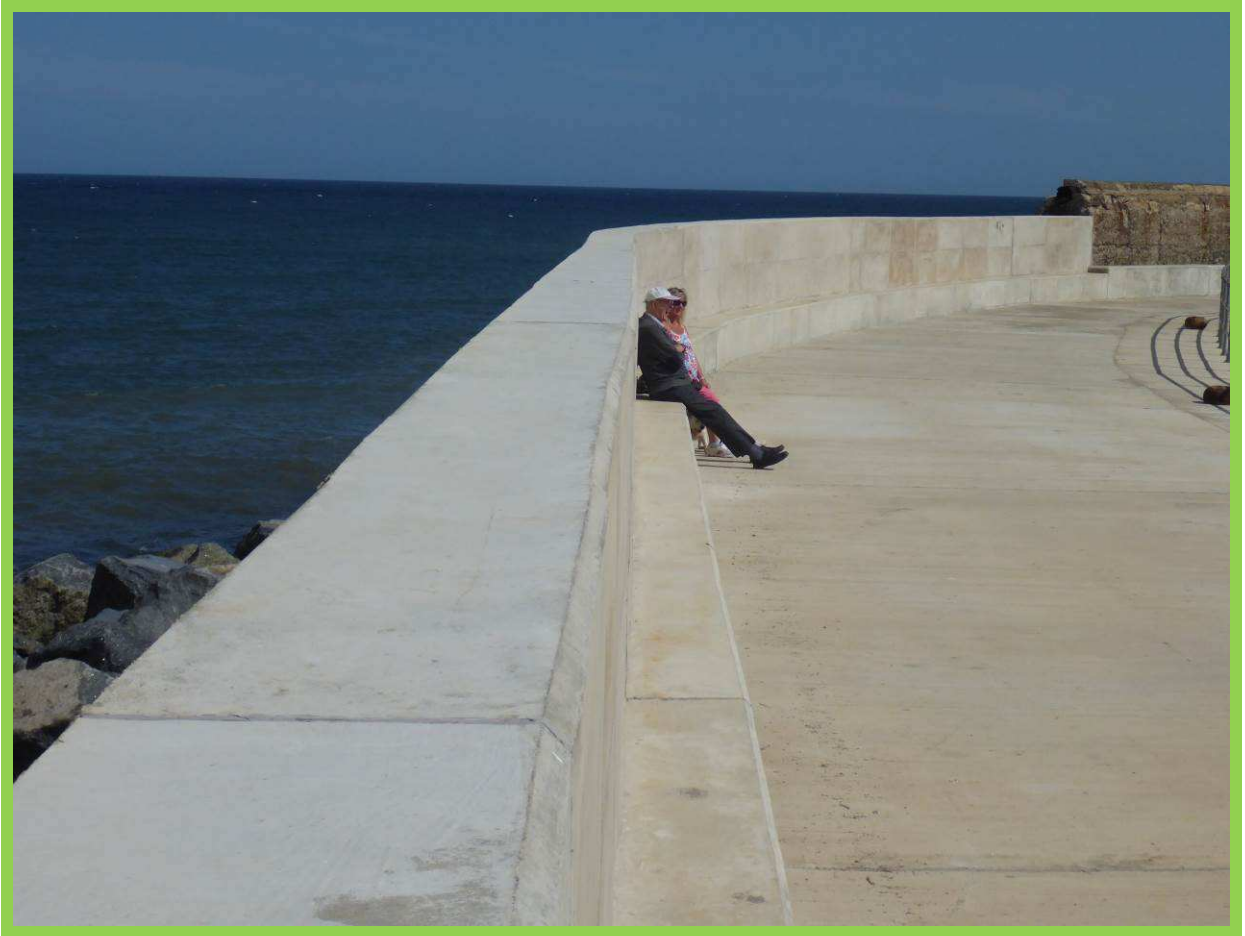
Rebuilt jetty wall (Asset Ref No. 1221D901D0201C02)
