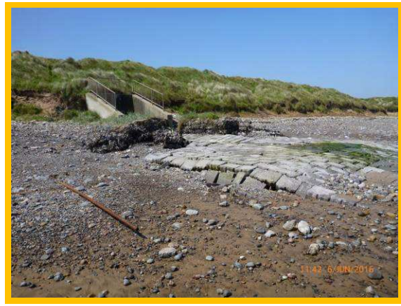
Concrete outfall structure (/C0701C01) CBU E52/10
