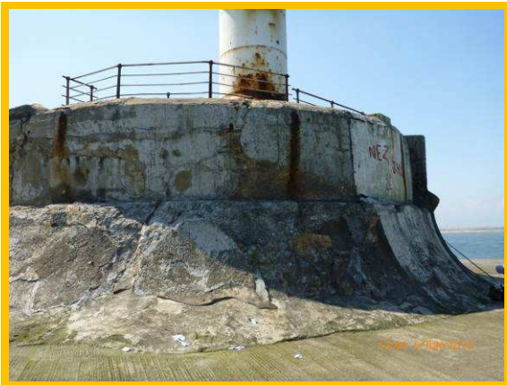
Northern extent of upper structure (/C0506C01)
