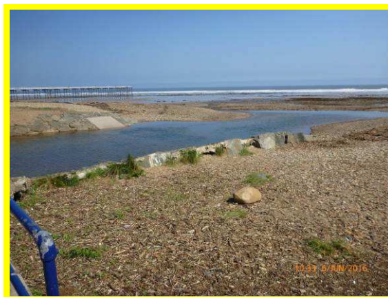
Exposed crest of grouted rock revetment (/C0704C06)
