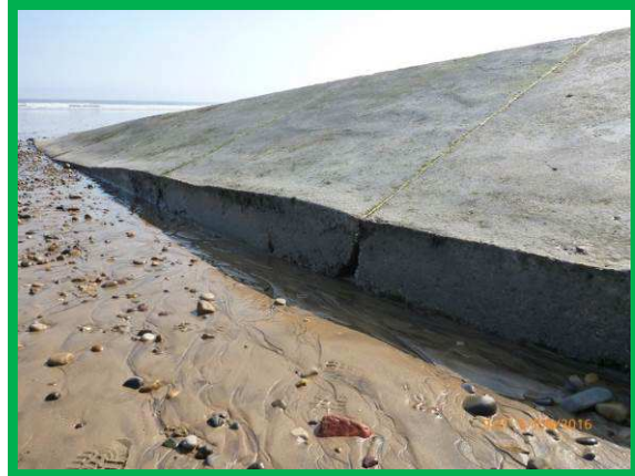
Western face of concrete slipway (/C0704C03)
