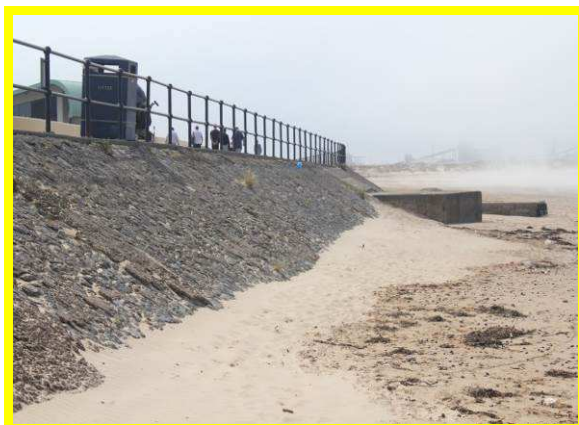
Grouted stone revetment (/C0601C01)
