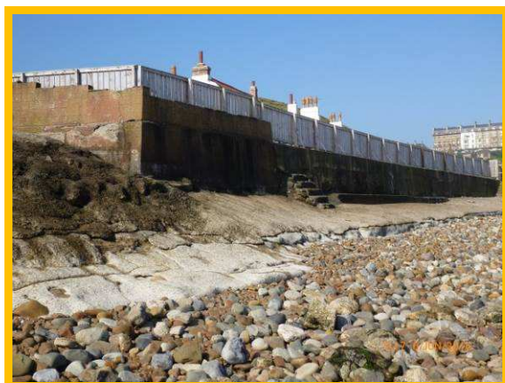
View looking west (/C0704C05)
