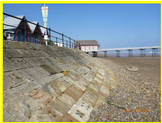
View looking north west (/C0704C01)
