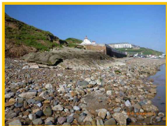
Undercutting/voiding in in situ concrete apron (/C0704C05)
