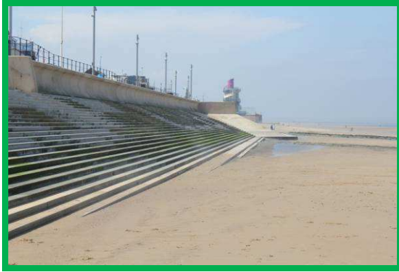
View looking north west – beach levels lower around access ramp and The Flashes rock outcrop (/C0602C01)
