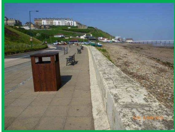
View looking west (/C0704C03)
