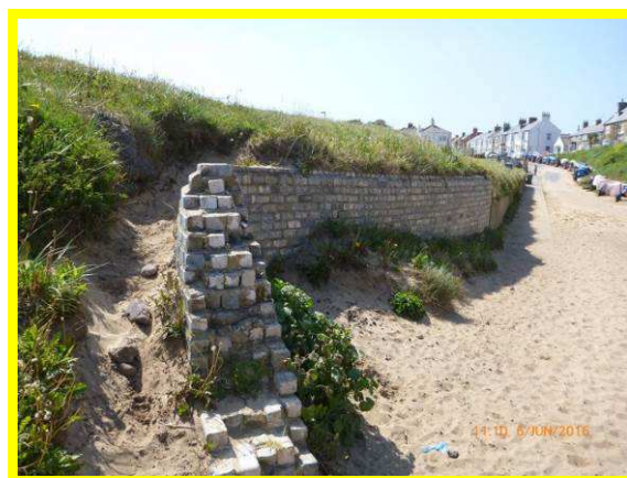
Masonry wall south east of beach entrance (/C0702C01)
