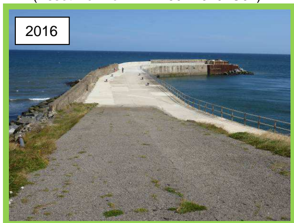
Repaired and improved structure in 2016 (Asset Ref No. 1221D901D0201C02)
