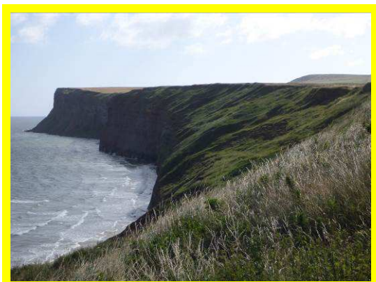
E53/3 to E53/1 Generally small scale slumping in the till layer of the cliff northeast of Saltburn (Locally Active except E53/2, right).
