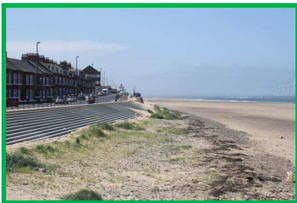
South eastern extent of stepped concrete defences (/C0602C01)
